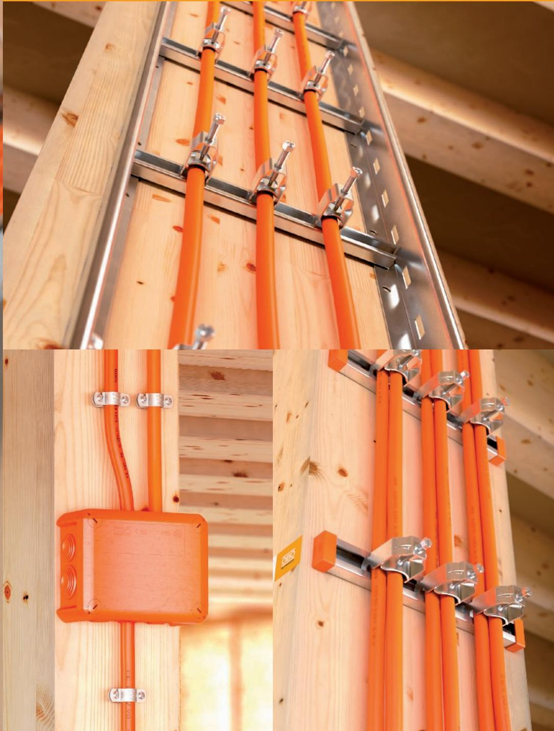
**1** Cable route under the beam in a lengthwise direction:
