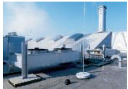
*Insulated lightning protection on roof fittings*
