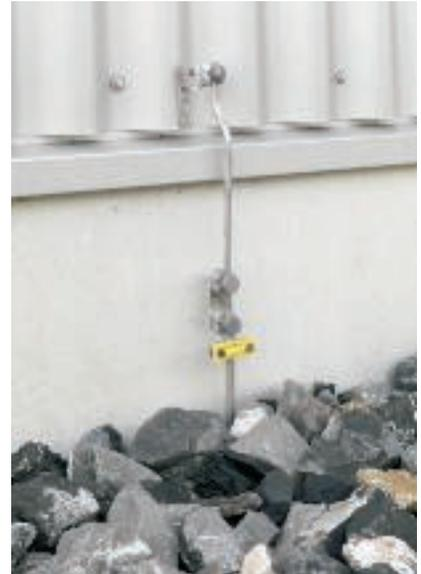
*Separation point in an earthing system plant*
