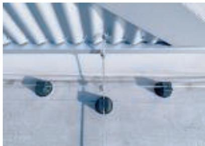
*A metal facade connected to the lightning protection system*
