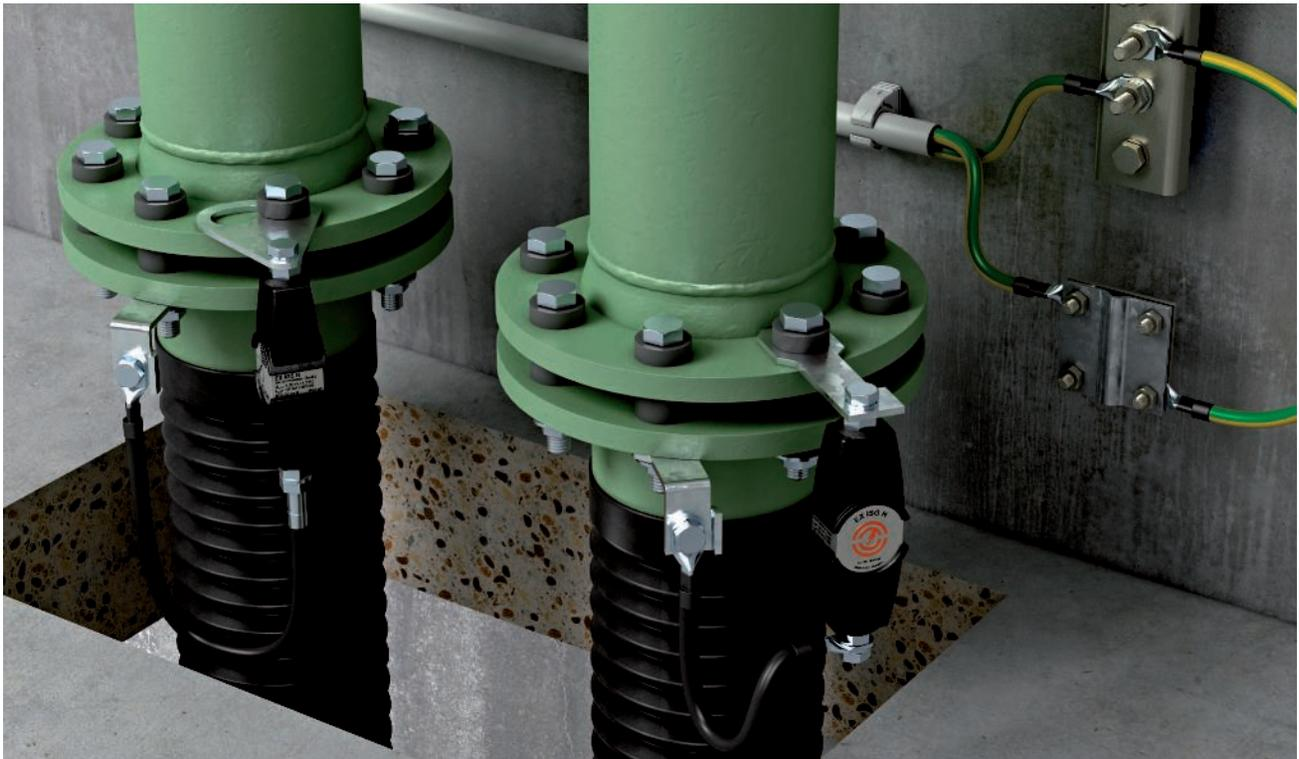
Spark gap mounted on insulating sections
