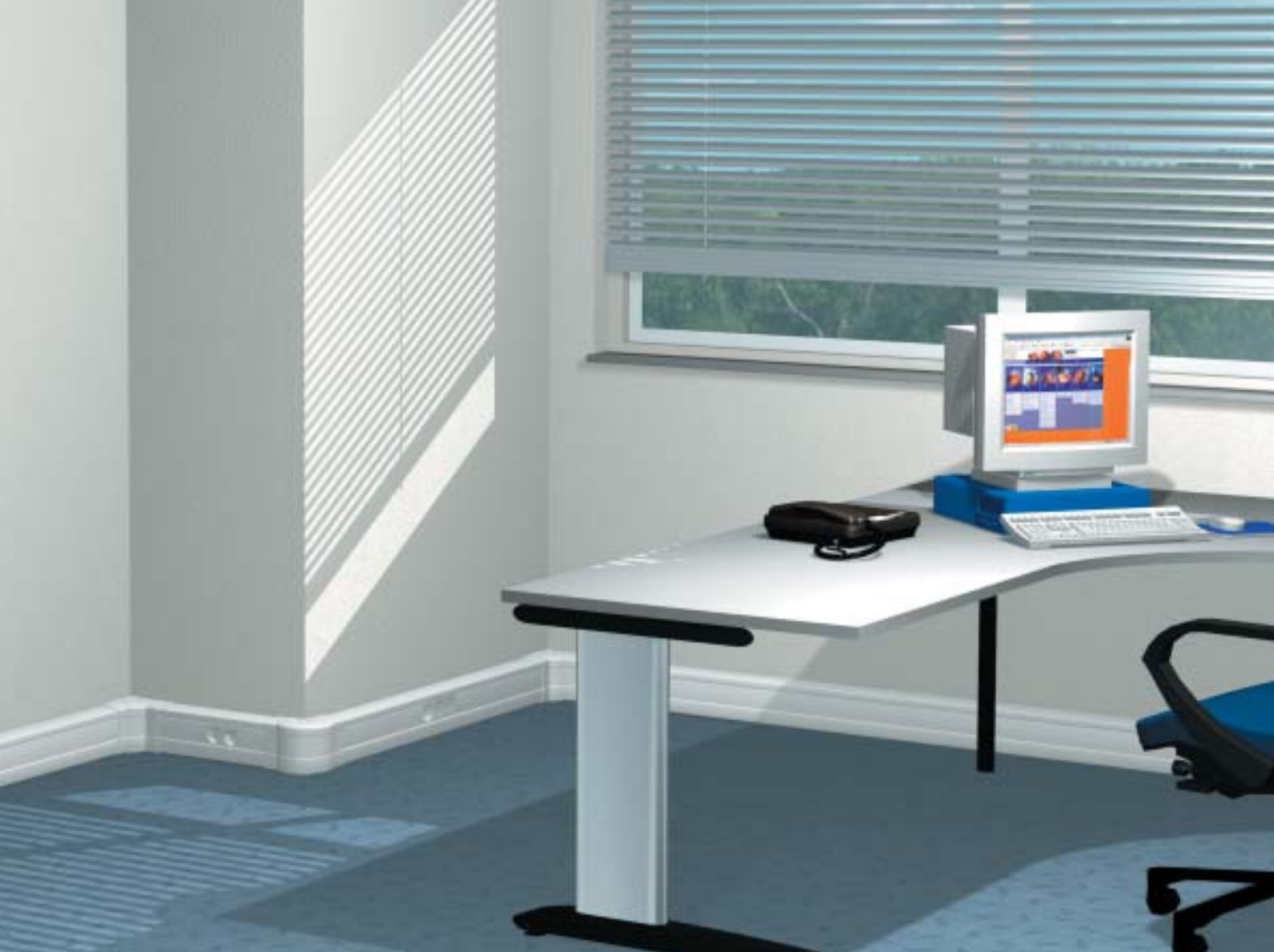
▲ Example 3: Rapid 45, height 100 mm Installation as dado rail duct
