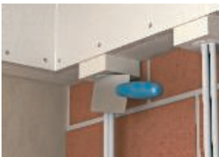
Filling of the cable exits
