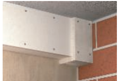
Wall connection for I 90 duct
