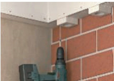
Preparation of cable exits
