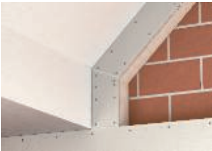
Use of variable duct routing
