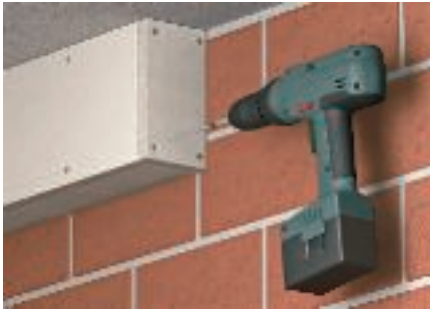
Mounting of end piece
