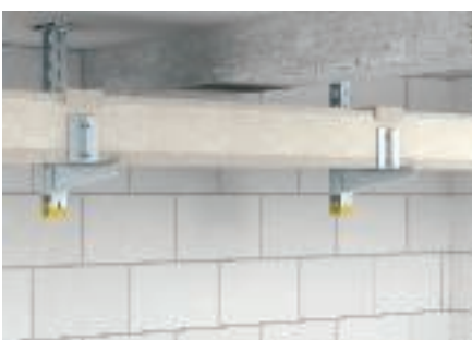
Mounted on OBO mounting systems to go under obstacles or for direct floor crossings.
